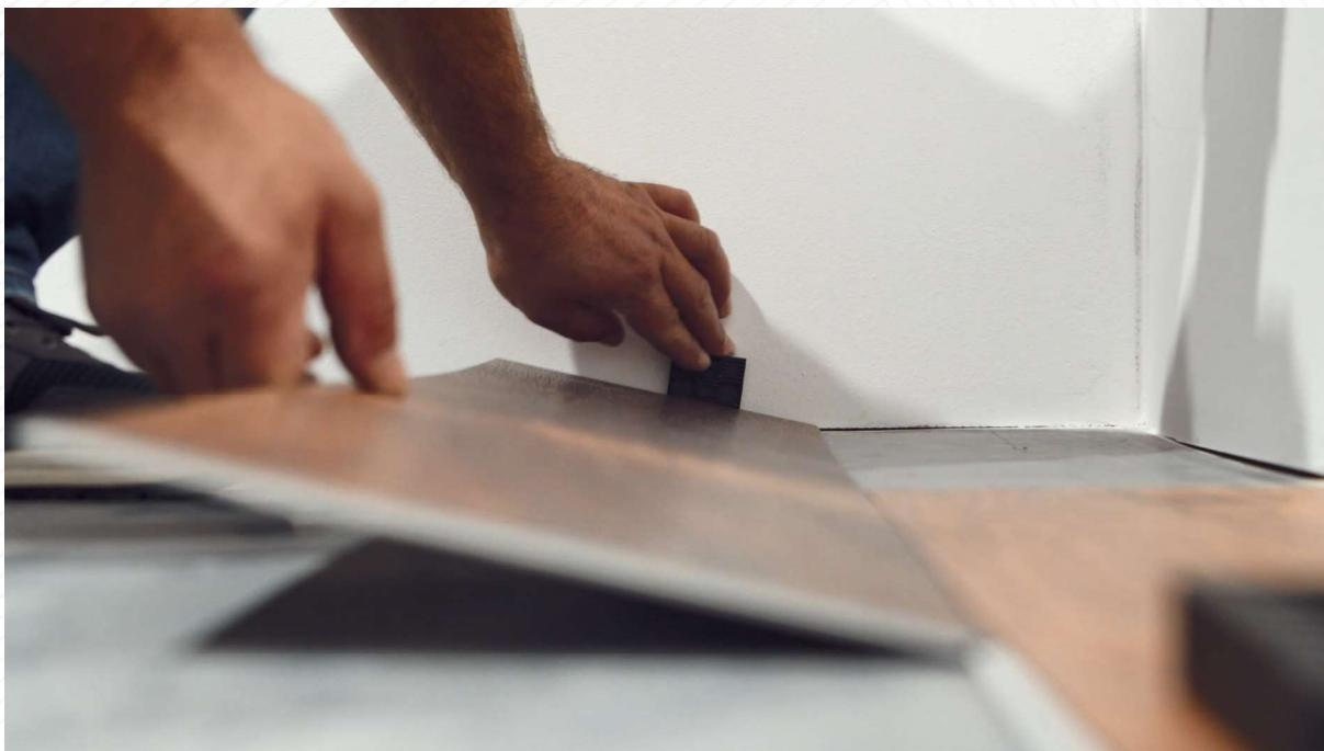
5. Start the installation by placing supporting planks by the wall, keeping the extension gap. You should place one supporting plank per each short seam of first row. Supporting planks will be removed in further installation steps.
