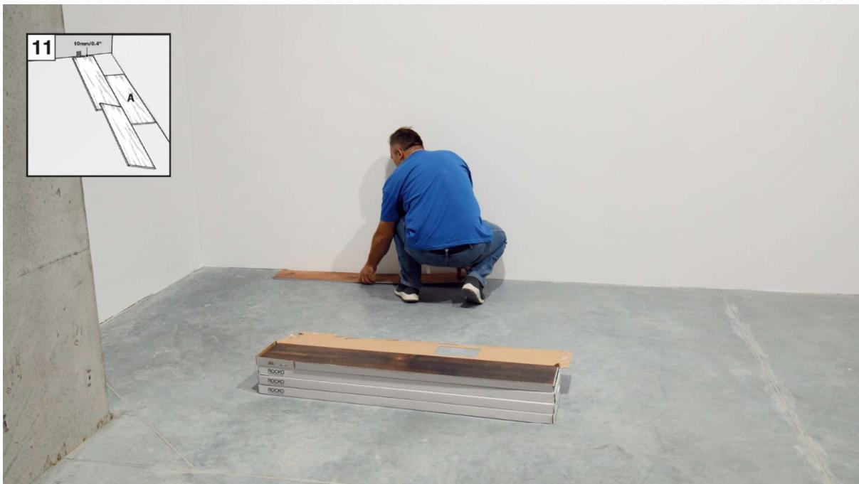
6. Start the installation at the left hand corner and proceed with the tongue facing the wall. When starting your first row, lock the two first planks in place by folding down second piece, then tap down on the top of the planks on the short seams using tapping block and a hammer.
