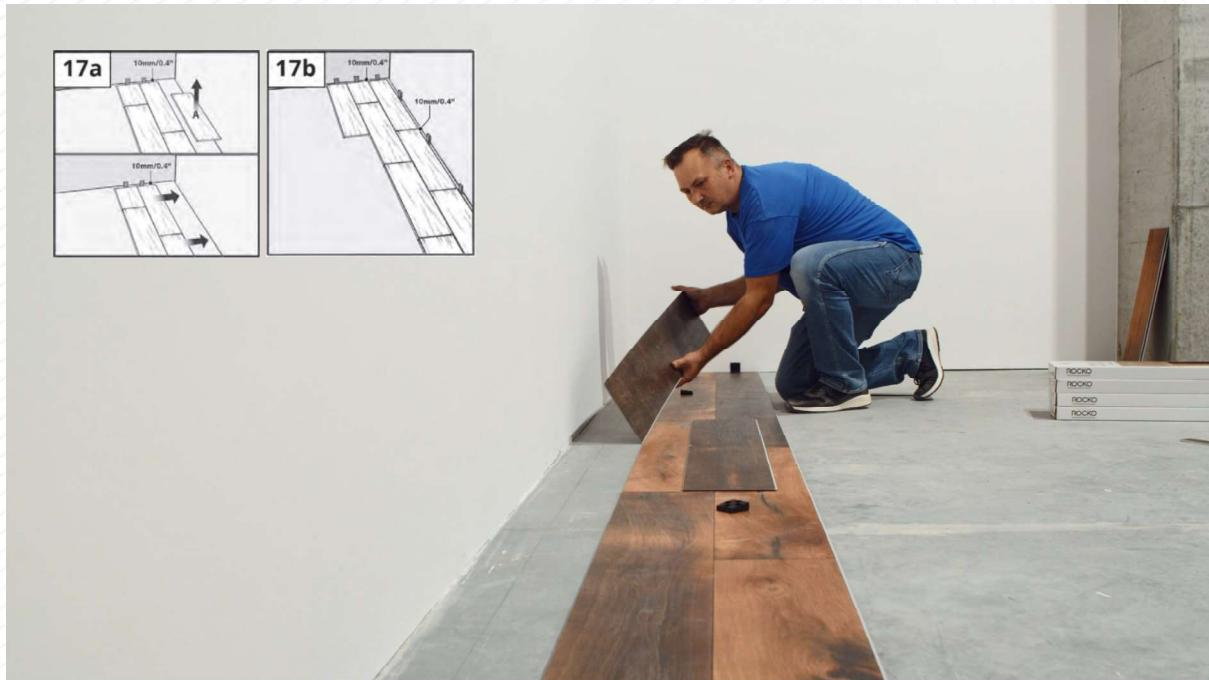
10. Continue the installation staggering the joints at least 40cm (16-in) and maintaining the extension gap – the staggered seams pattern can be repeated each row, or be random.
