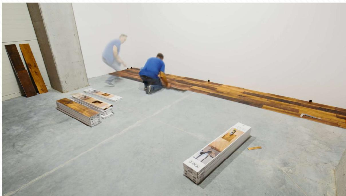
11. Cover the extension gaps by the Rocko skirting boards, installed at the end of the project.
