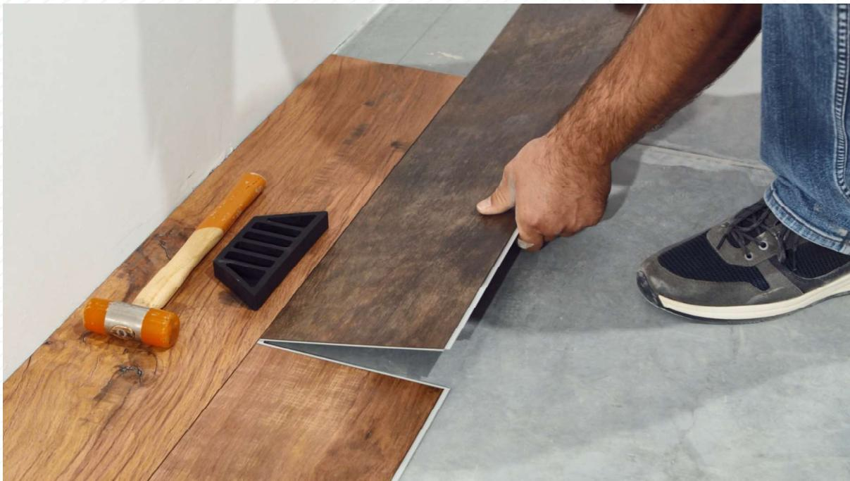
7. To cut the end plank in first row, simply mark the proper measurement and score the plank using utility knife and a straightedge, then just snap the plank along the score line. You will also need to back cut the underlayment on the bottom of the plank.
